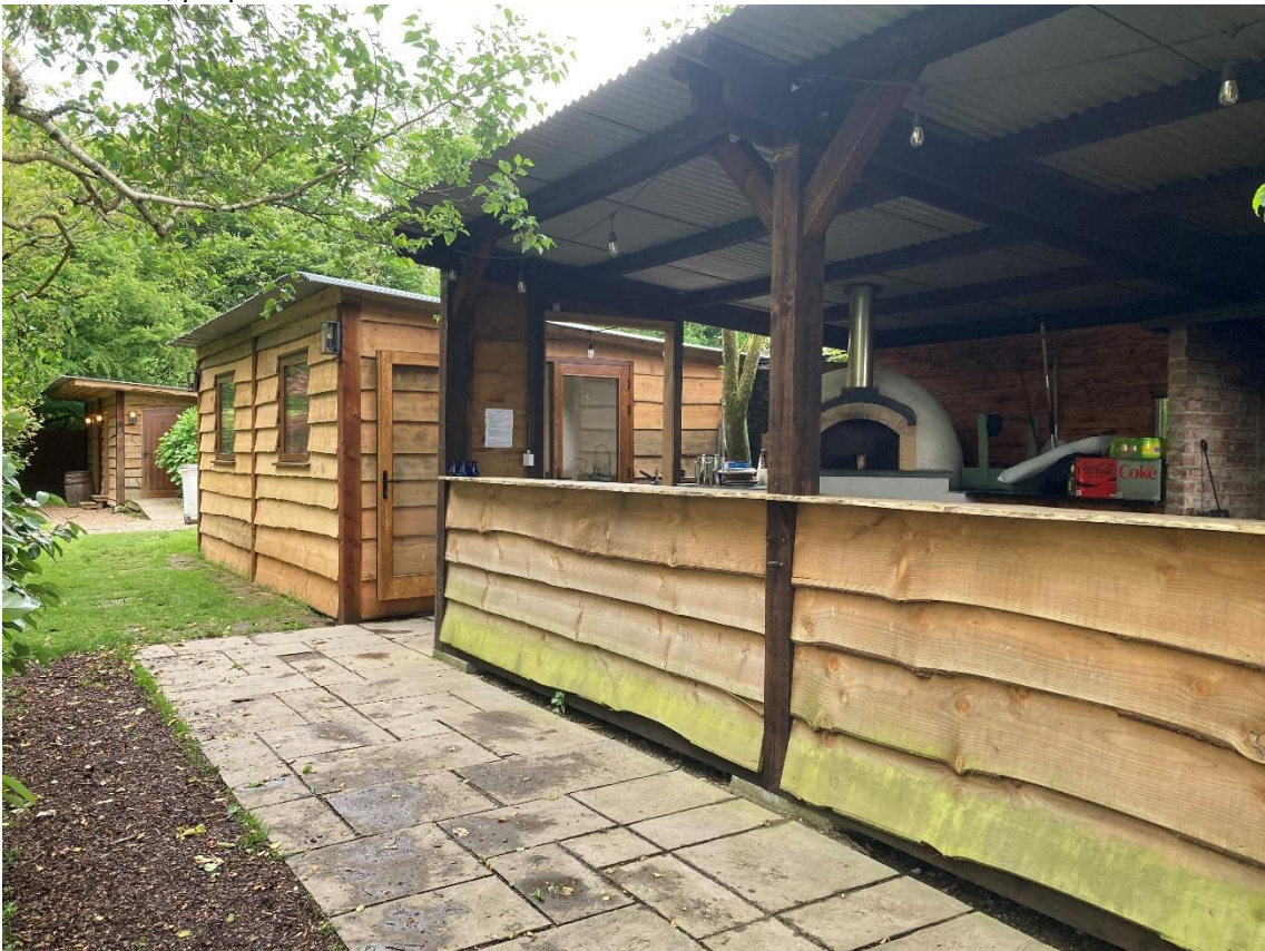
Fire kitchen, prep kitchen and toilet block
